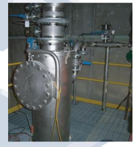
The concentrated non-condensable gases were then scrubbed using a mixture of demineralised water and sodium hydroxide. The gases were safely transported using a steam ejector and were incinerated in the lime kiln. The system was designed to also use white liquor as the scrubbing liquid.
